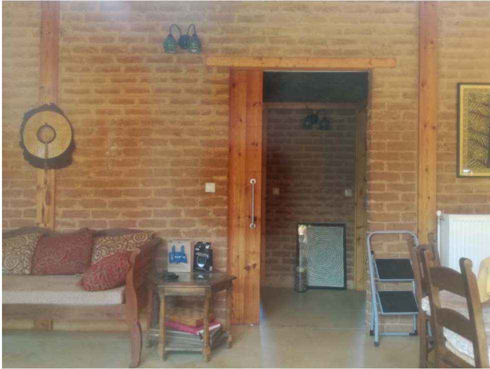
Figure 2.3: Interior wall made of adobe. European Sustainability Academy in the area of Apokoronas, Crete. Photo E. Frangedaki
