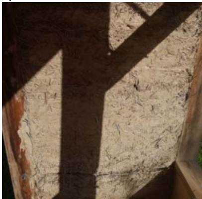
Figure 2.9: Light clay Structure by Piliko team (photos E. Frangedaki)
