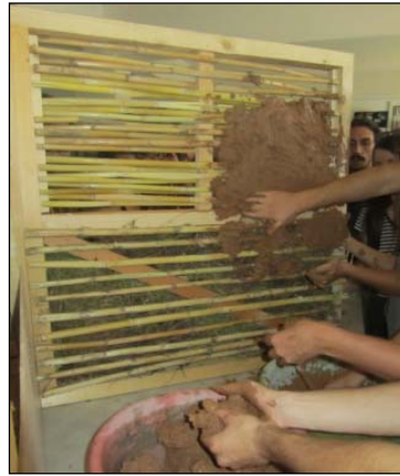
Figure 2.5: Wattle & Daub wall constructed in the laboratory of NTUA.
