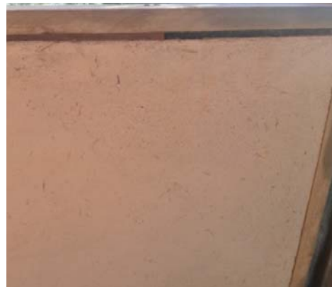
Figure 2.10: Light clay interior wall with mud plaster
