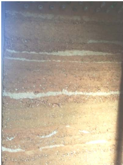
Figure 2.7: Rammed earth by Piliko team (photo E. Frangedaki)
