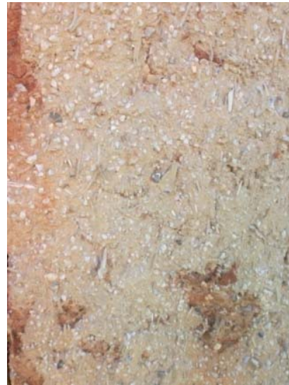
Figure 2.8: After 5 years without rain protection), Piliko team (photo E. Frangedaki)
