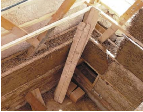
Figure 8.2 Wooden load bearing structure
