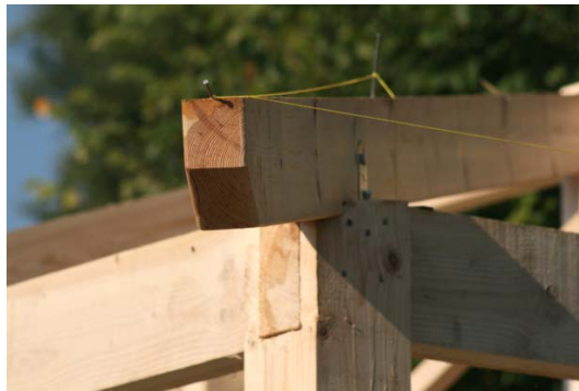
Figure 7.4: Wooden frame details
