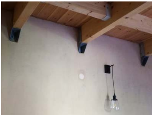
Figure 8.6 Interior, detail of the 1st floor
