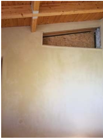
Figure 8.4 Interior earthen plasters
