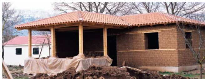
Figure 7.6: The mud house in Trikala, construction phase
