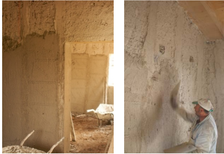
Figure 7.7: Plastering the adobe house
