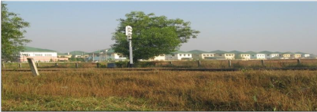
Plate 2. Khayaypin Yeikmon: Khayaypin Yeikmon 1 and Khayaypin Yeikmon 2 with modern-style two storey single houses, locating on Khayaypin Road in Chittigone Ward.
