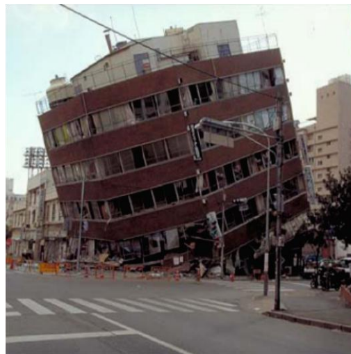
(b) Collapse due to Seismic Torsion
