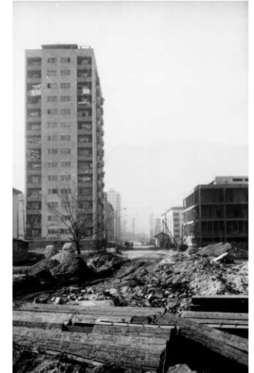
Tower in the residential settlement Karpoš 2 (left) and the Faculty of Technology (right). Source: Constantinos A. Doxiadis Archives. © Constantinos and Emma Doxiadis Foundation.
