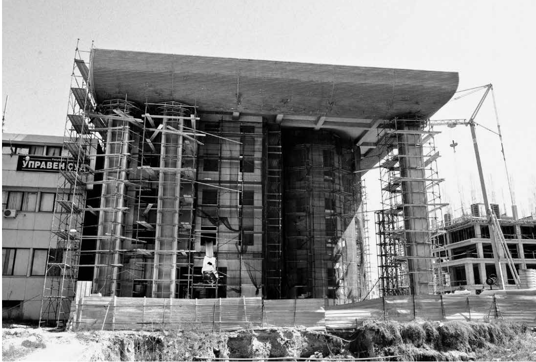
The MEP SO building under refurbishment. Photo: Maja Janevska-Ilieva.
