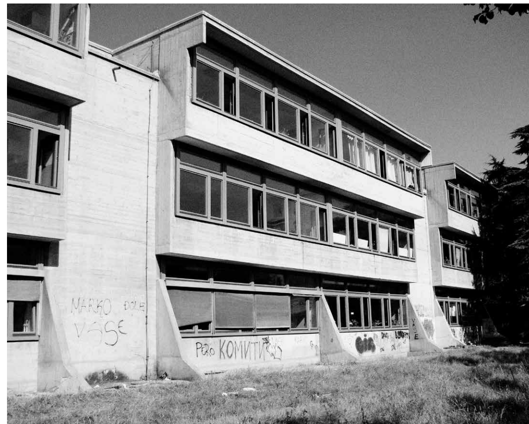
Elementary School "Johann Heinrich Pestalozzi", Skopje. 1967-69. Alfred Roth (1903-1998). Exterior view. Photos: Ana Ivanovska Deskova, 2009.
