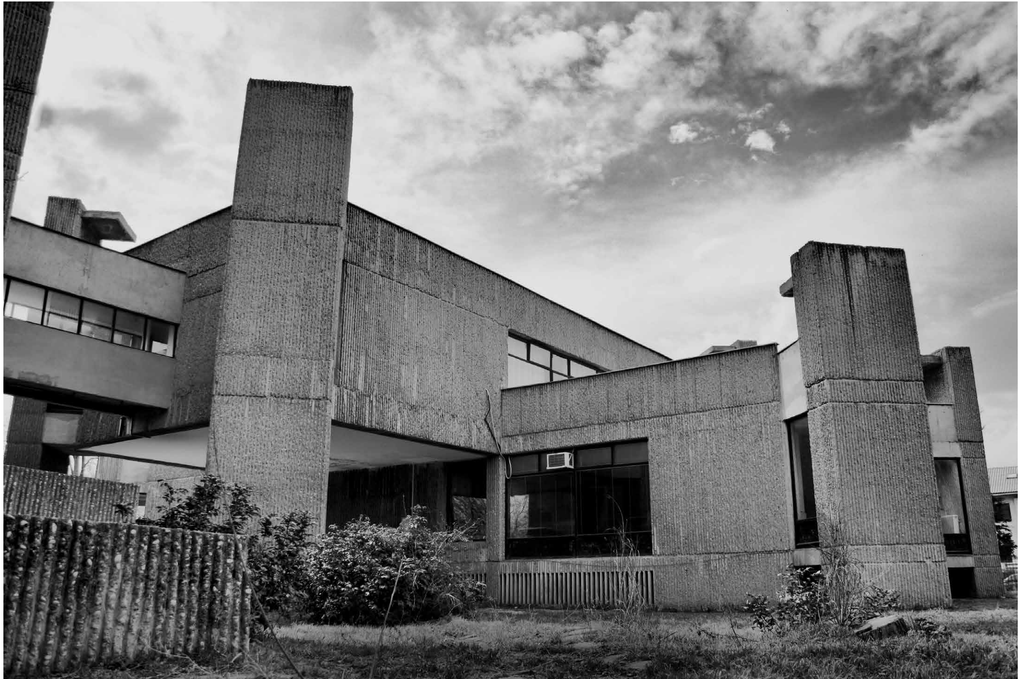
City Archive, Skopje. 1966–68. Georgi Kon- stantinovski (b. 1930). Exterior view. Photo: Damjan Momirovski, 2008.
