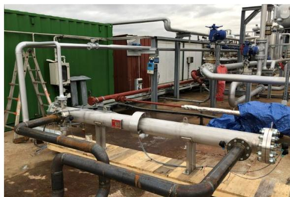
Figure 2: Test heat exchanger installed in Soultz power plant on 2019 (Ravier et al., 2019)
