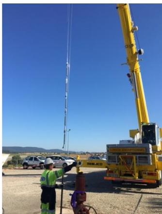
**Figure 3: Deployment of a fiber optic in a Soultz geothermal well by Febus Optics, September 2018**
