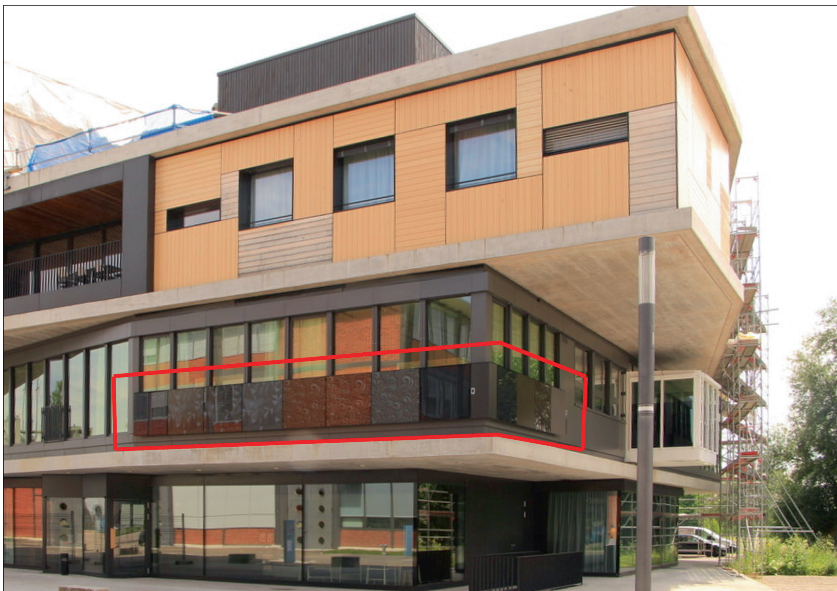
Figure 1: View of the NEST building from West with the 12 modules (red).
