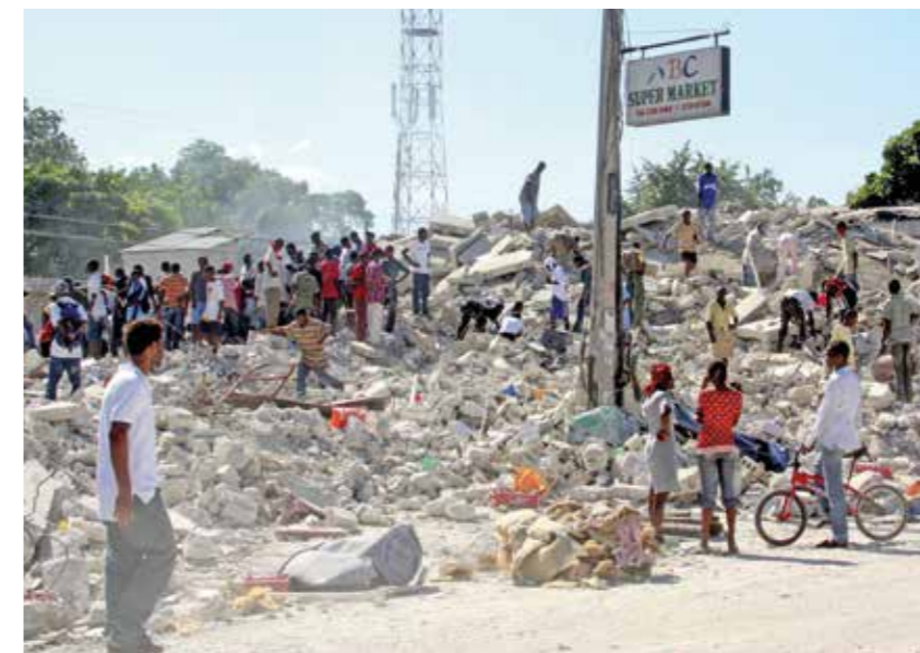
Figure 9.3 Collapsed supermarket in Haiti during earthquake of 12 January 2010. © UNEP
