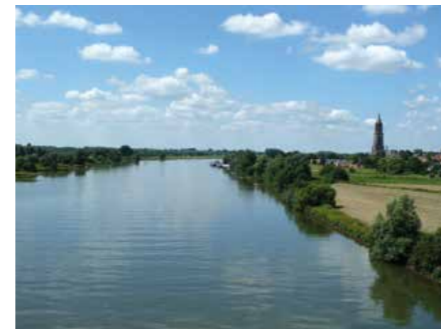
Figure 6.4 Nederrijn River Rhenen, Netherlands. © M. van Staveren
