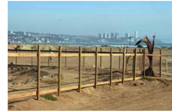
Figure 4.3 Left: Fore dunes in Chile that serve as buffers and protect from wind and waves. These fore dunes have been partly removed to create space for coastal infrastructure. The new infrastructure will now be directly exposed to storms and waves and even tsunamis that occur along the central Chilean coast. Right: Destruction of coastal dunes in central Chile. © U. Nehren
