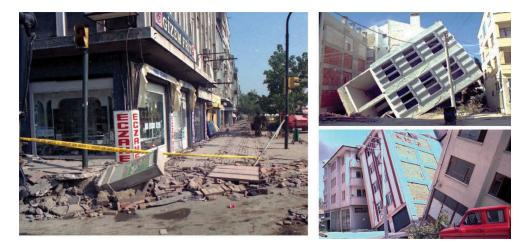
Figure 1. Typical photographs for buildings with Liquefaction Induced Damage (LID) (Provided by Adapazari and Sakarya Municipalities)
