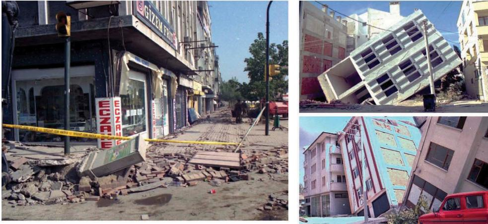
Figure 1. Typical photographs for buildings with Liquefaction Induced Damage (LID) (Provided by Adapazari and Sakarya Municipalities)
