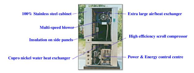
Figure 10. GSHPs extract solar heat stored in the upper layers of the earth
