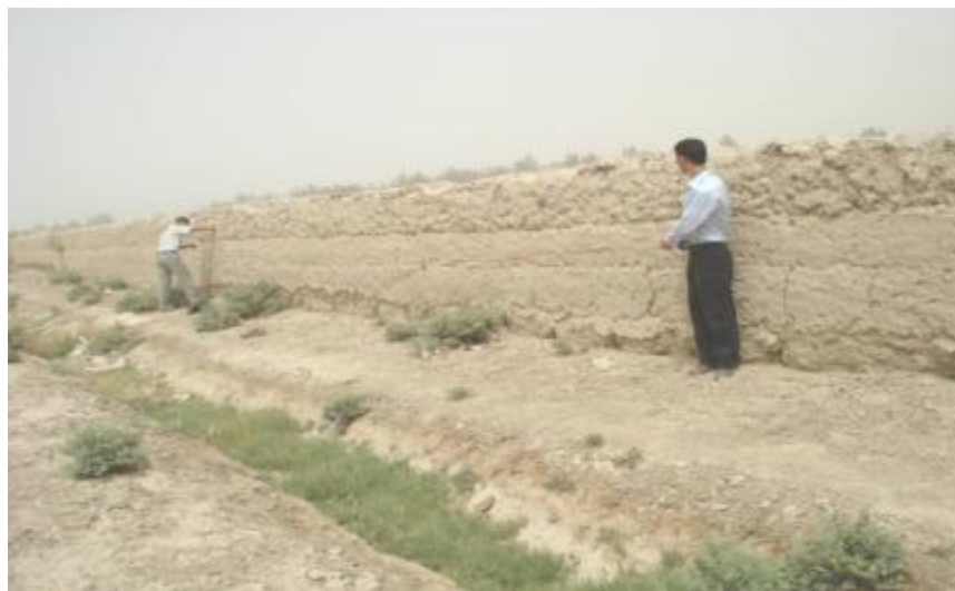
Fig2: View of Mud wall wind break which was used in this study as an abiotic windbreak
