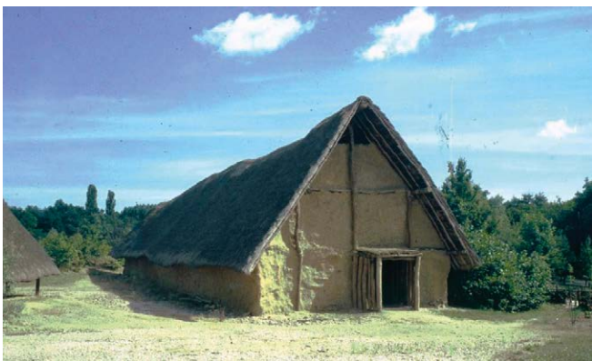
Figure 6. A reconstructed typical LBK house. The walls are made of adobe. Silty (loess) soils associated with straw provide excellent material for such construction.
