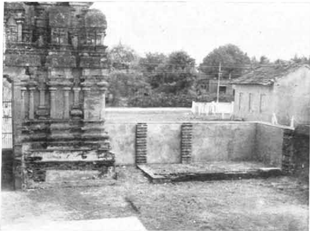
B. Nedungadu : Siva temple, after conservation. See p. 86
