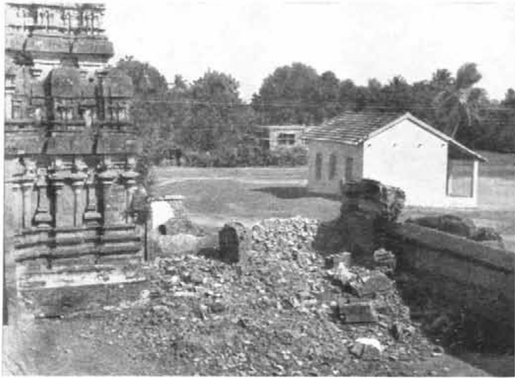
A. Nedungadu : Siva temple, before conservation. See p. 86
