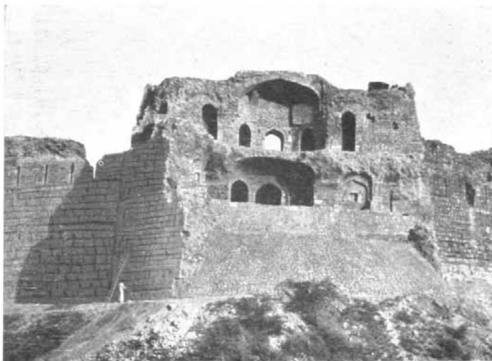
B. Delhi : Purana Qila, after repairs. See p. 84
