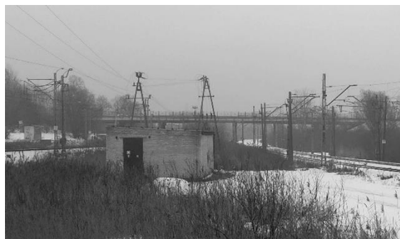
Figure 6. View of the energy installation near the railway viaduct – national road No. 15 over lines No. 353 and No. 281
