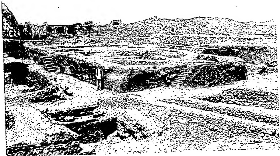
(b) CROSS-WALLED STUPA IN BLOCK E', FROM SOUTH-EAST.
