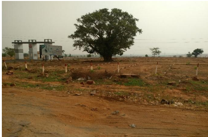
Image 9: The under construction Shine city on SH-5 surrounded by Marihan forest range
