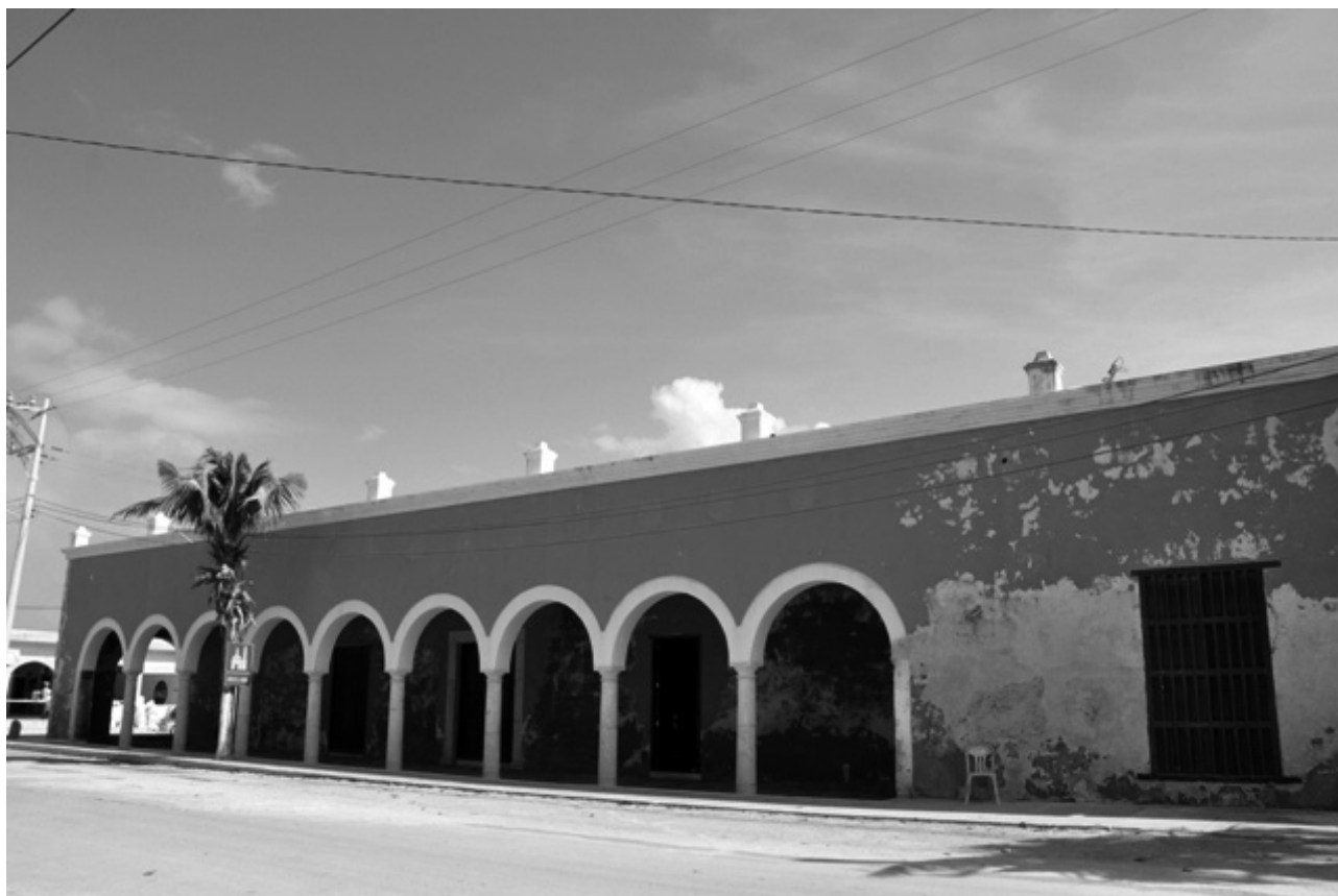
FIGURE 1. HISTORICAL BUILDING LA ADUANA IN SISAL, YUCATAN
