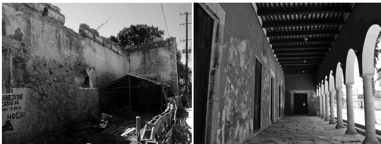
FIGURE 2. LA ADUANA: BEFORE (LEFT) AND AFTER (RIGHT) RESTORATION
