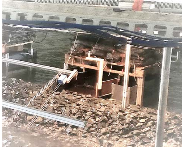
Figure 2-3. General layout at the entrance of an overtopping reservoir (run-up wave gauge and acoustic wave gauge to identify overtopping events).
