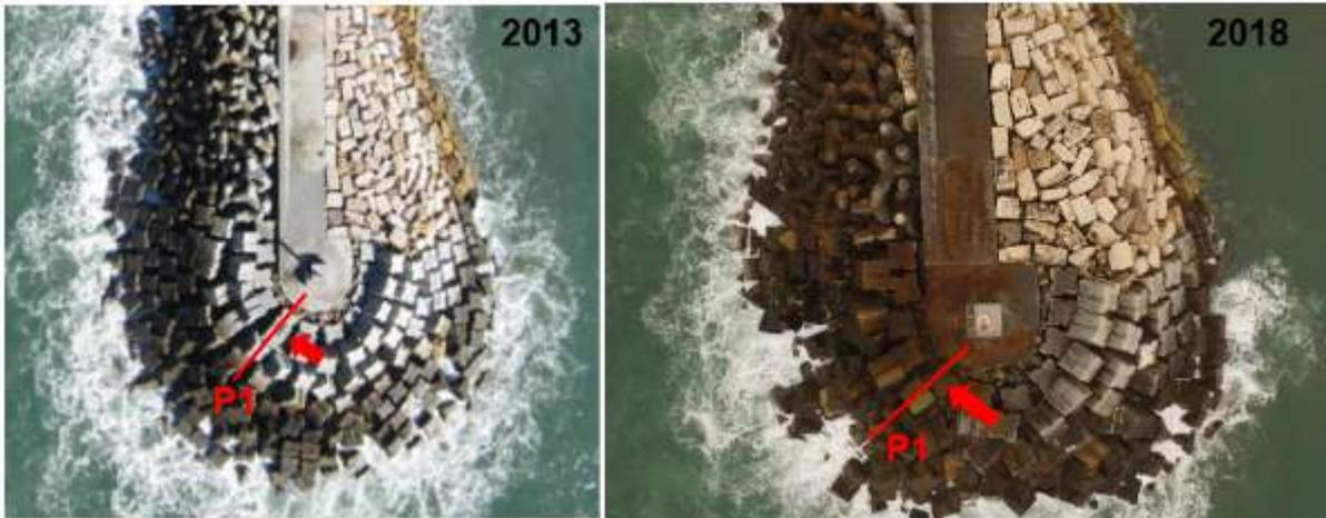
Figure 11 - Aerial photos of Ericeira's breakwater in February 2013 and April 2018. Definition of a vulnerable section (P1)
