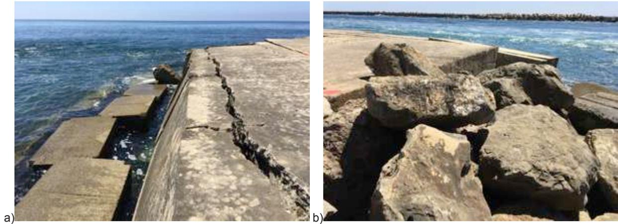
Figure 6 – Faro-Olhão’s west breakwater – Sections with problems (see also Figure 3b): a) Point 12 (section C, interior); b) Point 15 (section C1, exterior)
