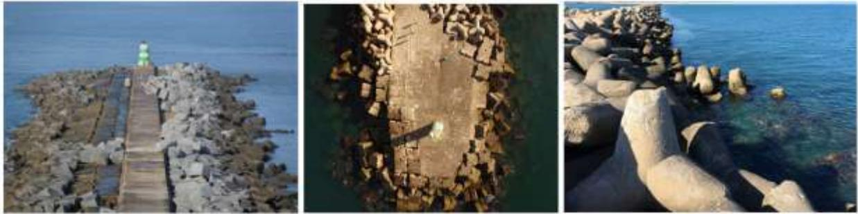
Figure 1 - Signs of fatigue of the elements and materials in rubble-mound breakwaters
