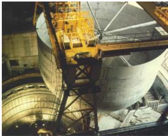
Figure 1: Arrival of the safety vessel inside the reactor pit of Superphenix
