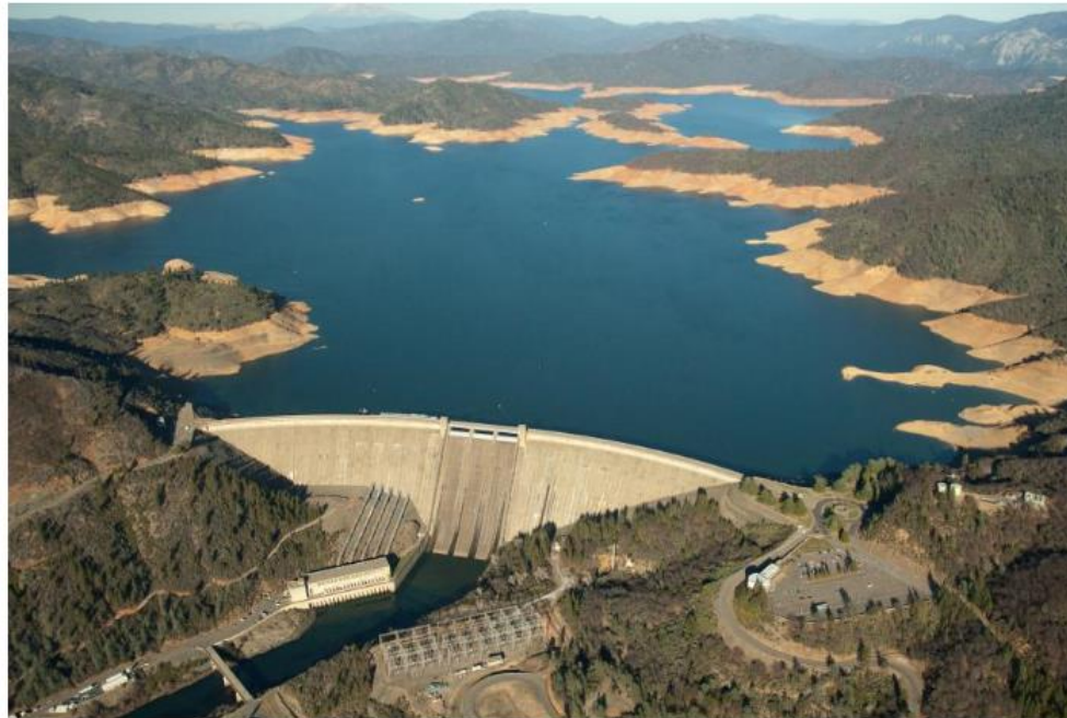
Aerial view of low water level in drought conditions at Lake Shasta in California, 2014. DWR (Department of Water Resources), California.
