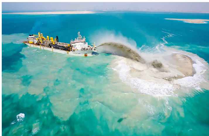
Fig. 4.46. Soil jetting for the formation of a new island [7]
