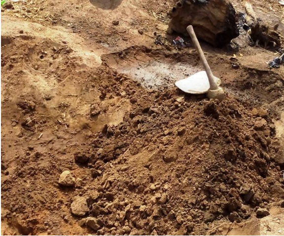
Plate 7. Bad tillage of top soil to mould block for housing
