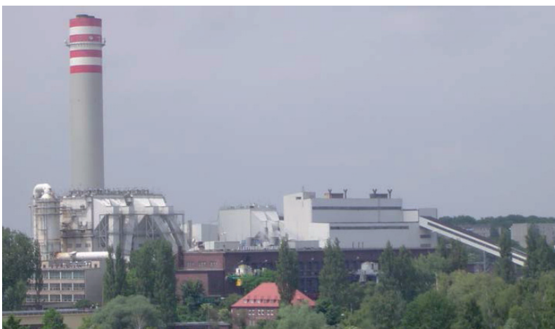
Fig. 6.30. View of Pomorzany Power Station – flue gas humidifier tower of EBFGT plant
