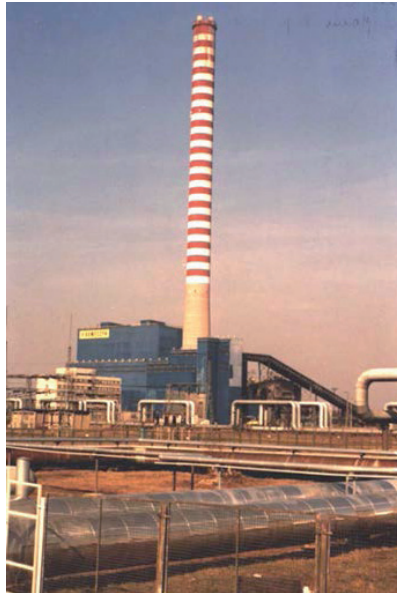
Fig. 6.2. General view of Kawęczyn Power Station
