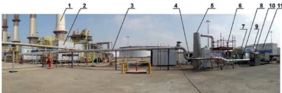
Fig. 6.19. General view of the pilot plant at the Jeddah Refinery: 1 – stack of boiler, 2 – boiler, 3 – flue gas duct, 4 – pilot plant control room, 5 – gas conditioning column, 6 – pilot plant stack, 7 – cartridge bag filter, 8 – thermal insulated duct, 9 – cyclone, 10 – ammonia dosing unit, 11 – mobile accelerator unit
