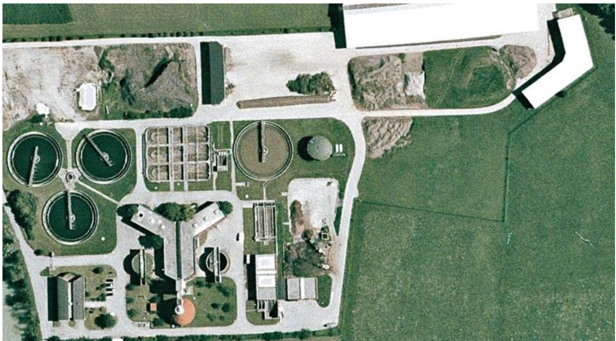
Figure 27: State of the WWTP Kirchbichl in the year 2000
