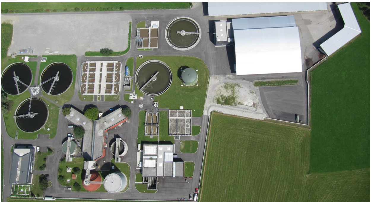
Figure 29: State of the WWTP Kirchbichl in the year 2015
