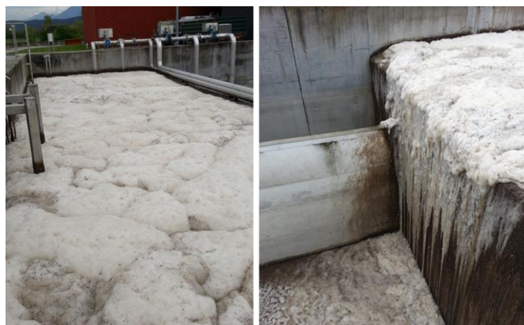
Figure 39: Foam formation in the SDE treatment tank Kirchbichl
