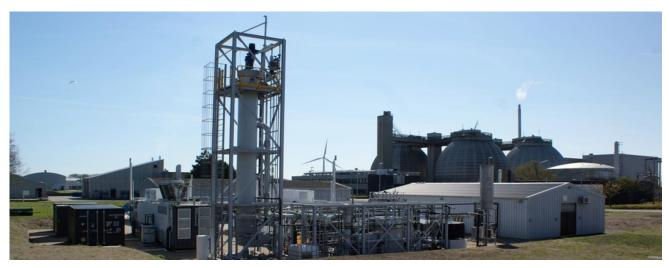
Figure 5 - View of the BioCat plant showing the reactor (left), balance of plant (center) and the biogas plant (background)
