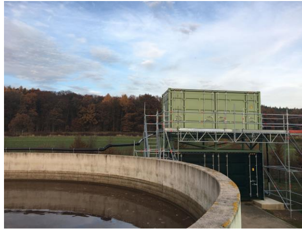
Figure 18: POWERSTEP microscreen plant in the Westewitz WWTP with SBR reactor
