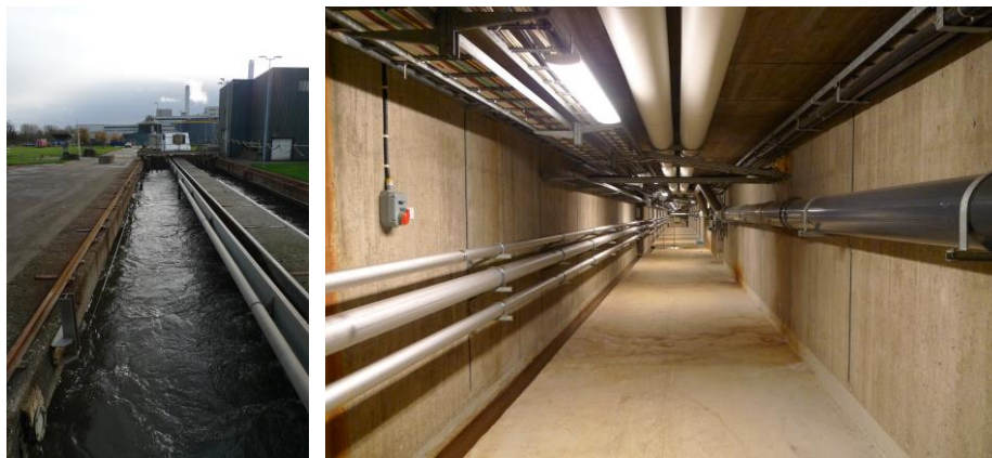
Figure 29: Grit chamber effluent (left) and pipework towards the Discfilter plant (right)
