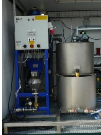
Figure 23: Polymer station
