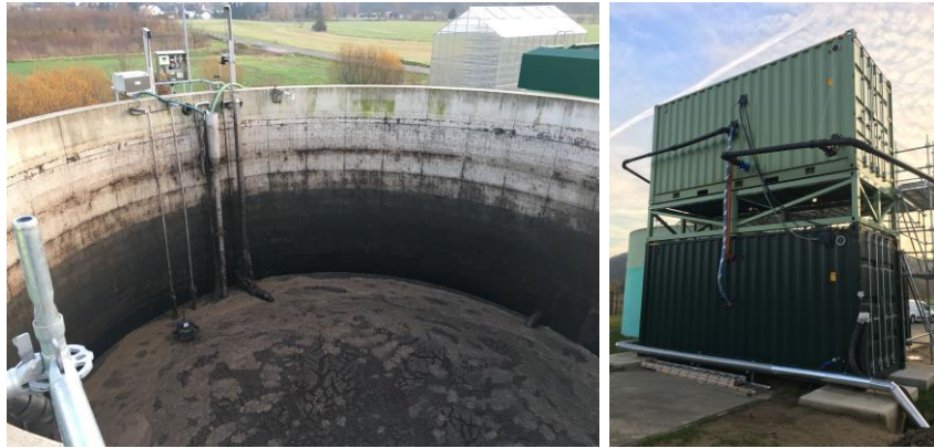
Figure 21: Sludge storage tank and piping connections at the Westewitz WWTP
