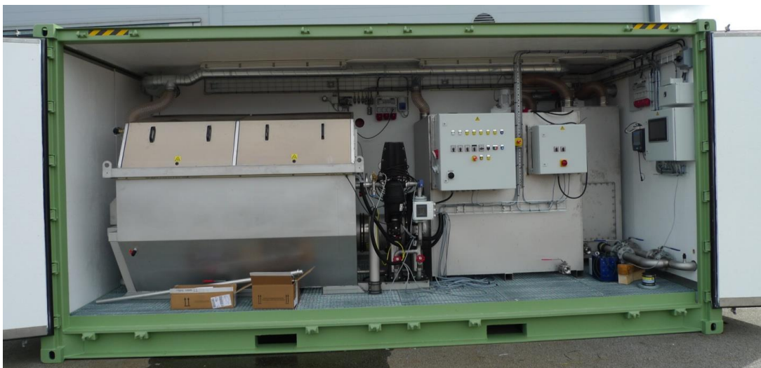
Figure 19: The filter container at Westewitz WWTP, with coagulation tank, flocculation tank, drum filter and control cabinets.
