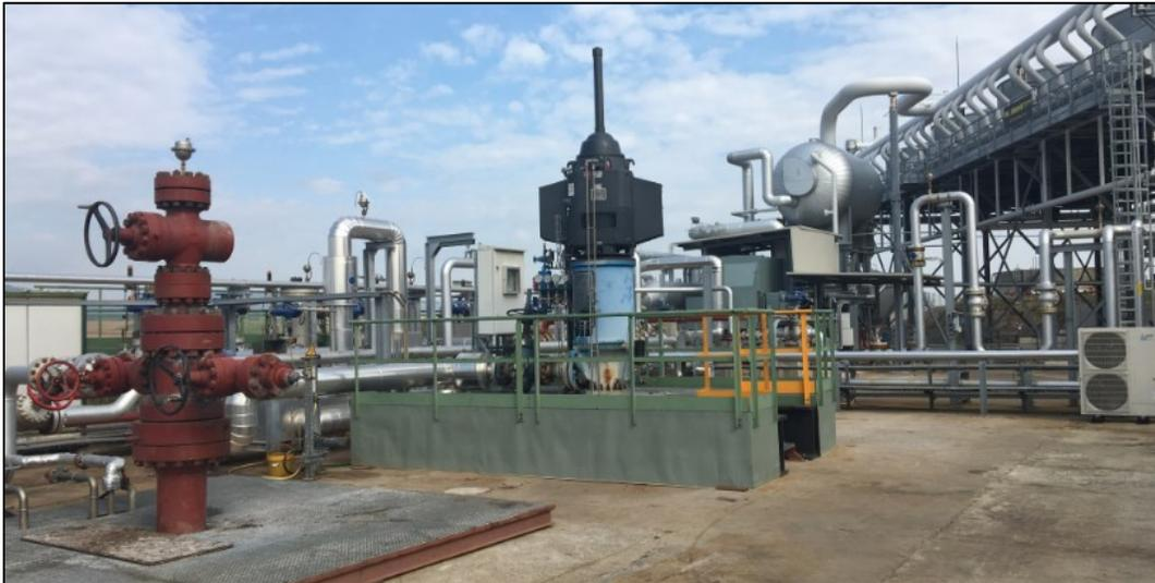
Figure 3: The Soutz-sous-Forêts power plant. On the left, the reinjection well GPK-3 well head, in the middle the GPK-2 production well head with the down-hole pump motor, and on the right the PORC plant. Credit photo ESG.
