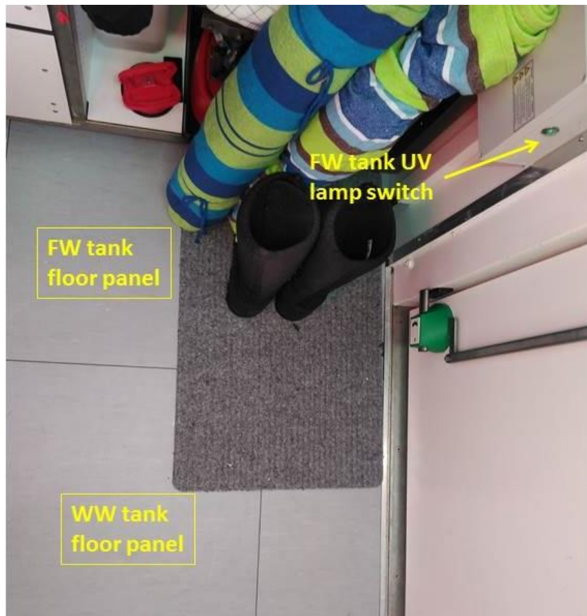
Figure 1: Cold porch with fresh and waste water tanks, and the lamp switch, position
