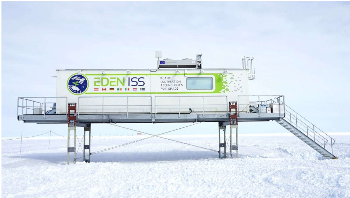
Figure 5: EDEN ISS facility following the elevation of the platform and installation of the platform stairs.
