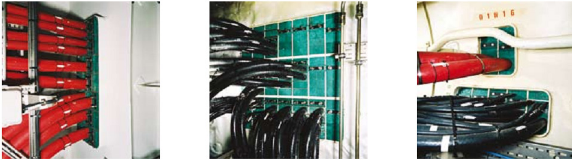
Figure 3-8: GK-Packsystem is used on ships to create water and gas tight connections through walls.
