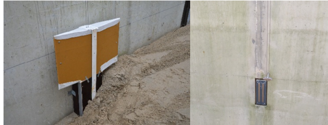
Figure 3-1: Box cover around reference electrode (left) and wires of resistance wave gauge and reference electrode below (right)
