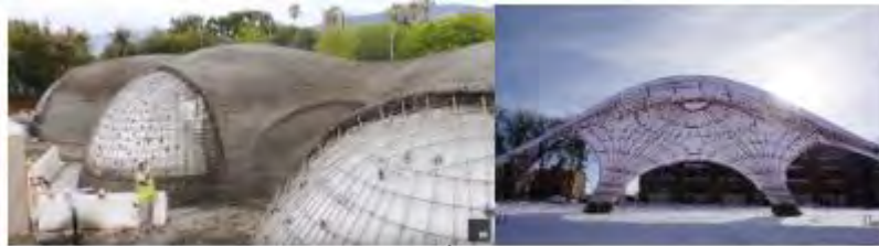
Figure 1. (a) Bini Shells withinflatables covered by a metal mesh as lost reinforcement to be sprayed manually with shotcrete. (b) Spray ice on fabric formwork and active bending metallic elements. "Zero bending moment" Lancelot Coar Winnipeg, Canada 2016.
