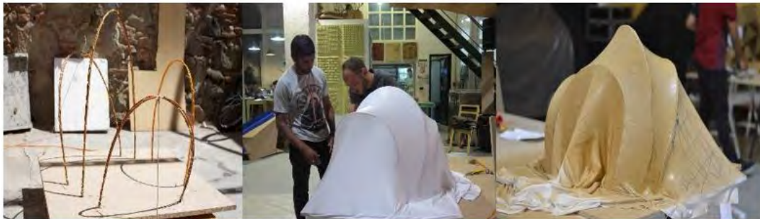
Figure 9. (a) Placement of the 3 peripheral and one middle arch materialized by a cluster of 2 or 3 0.3 mm diameter reeds. (b) Placement of lycra fabric stretched over the different arches. (c) First liquid clay mix robotically applied on the fabric and reeds formwork.
