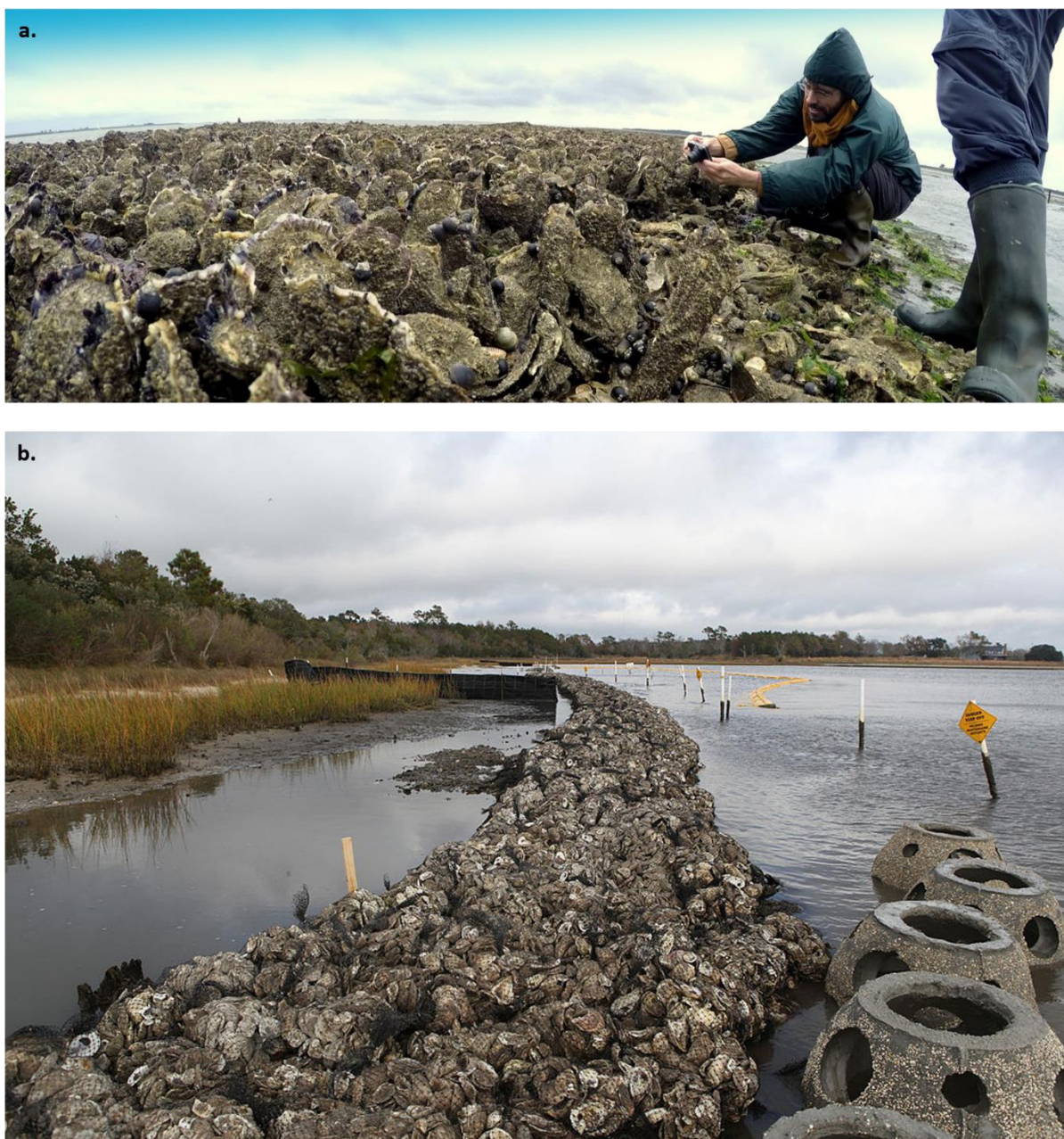
Figure 6 Oyster shell ecosystem services. a. An artificial oyster shell reef in the Oosterschelde (The Netherlands), acting as a settlement substrate for oyster larvae to promote reef growth with the secondary benefit of localised coastal erosion and sea level rise protection (Licence: Public domain, Credit: James Morris). b. An oyster reef constructed from oyster shell bags and shell aggregate reef balls along a segment of the North Carolina (USA) Shoreline. The reef protects the coast from erosion and promotes a healthy natural ecosystem (Licence: Public domain, Credit: Jackeline M. Perez Rivera).
