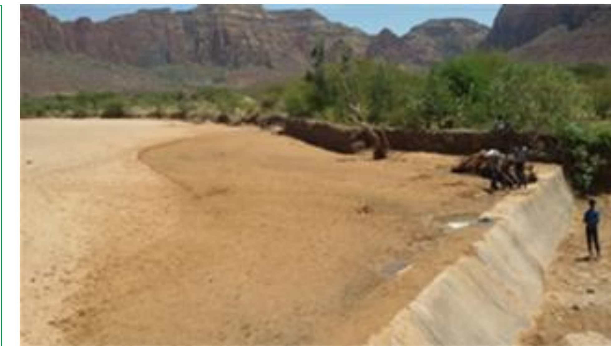
May Gobo sand dam
