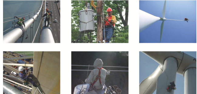
Fig. 1. Application scenarios in which aerial manipulation might be helpful. Left column: bridge inspection; central column: high-voltage electric lines inspection and fixing up; right column: rotor blade repairing.
