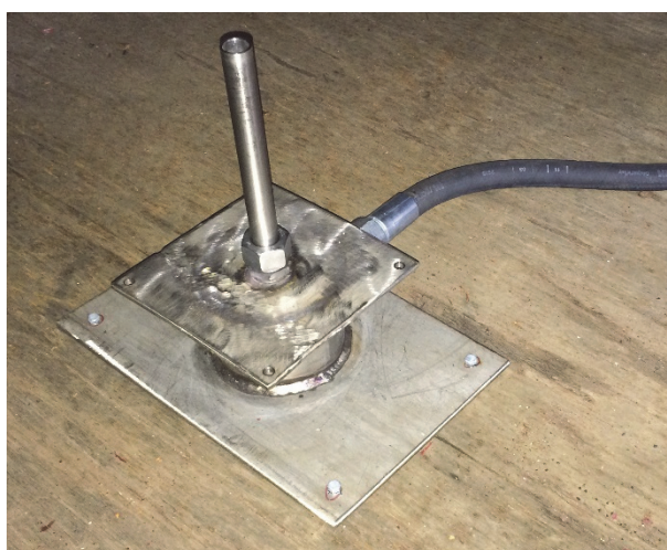
Figure 12: Pipe used for vertical jet release.
