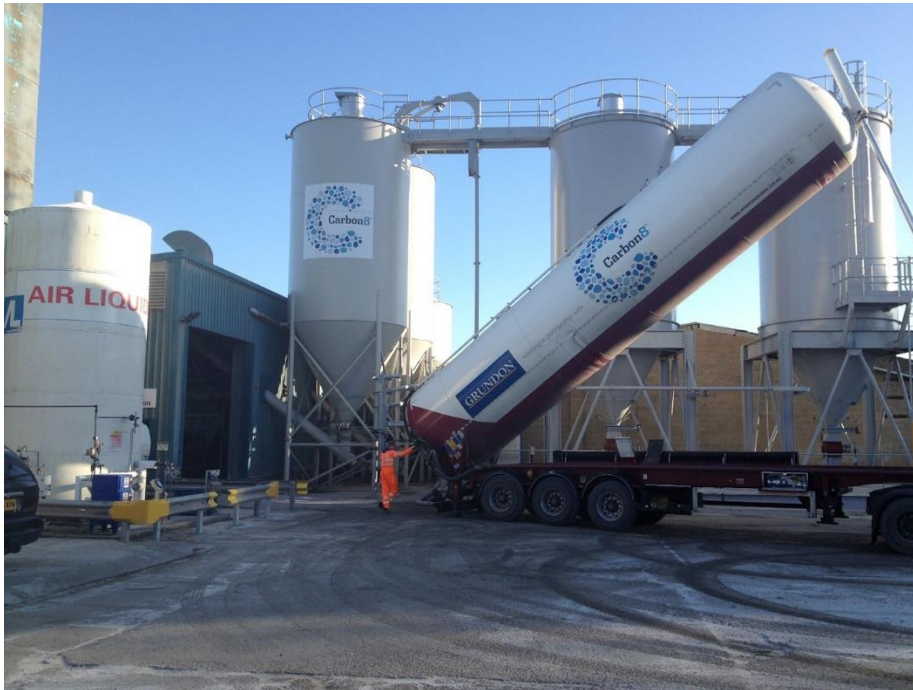
Figure 3-3 Carbon8 aggregate plant at the Lignacite site in Brandon, UK. Source: [22]
