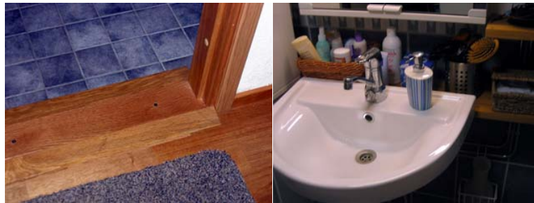
Figure 3. Ed's oaken thresholds (left) and integrated bathroom accessibility (right).
