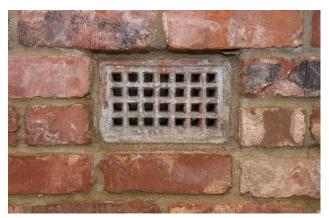
Figure 5: The air vent and surrounding brick work.
