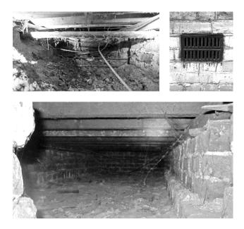
Figure 1: Images of typical voids and an air vent.
