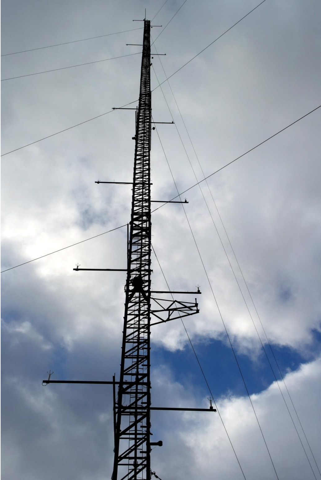
Figure A6 The mast showing the six measurement heights
