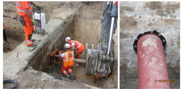
FIGURE 7 : PASSAGE DE CANALISATION AVEC JOINT ANNULAIRE
