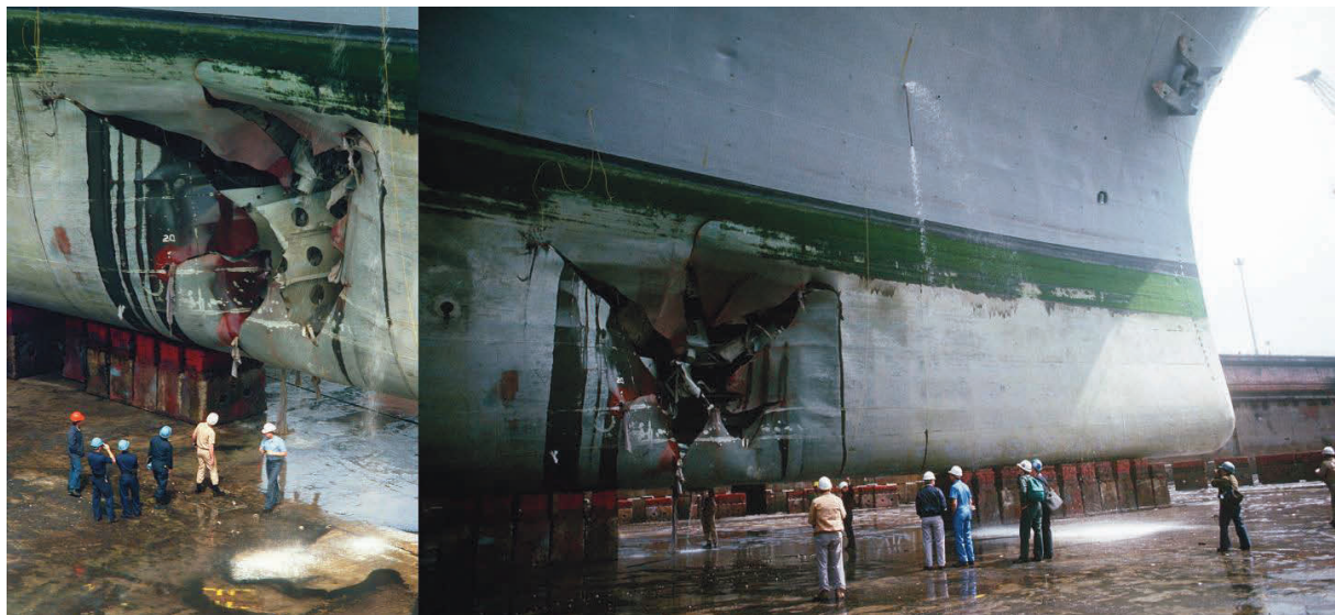
Figure 3 - Damage sustained by USS Tripoli during Operation Desert Storm (1991) due to a naval mine. Image reproduced from Nav Source (2018)
