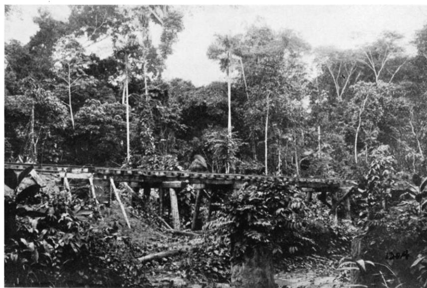
TEMPORARY TRESTLE, MADEIRA-MAMORE RAILWAY
