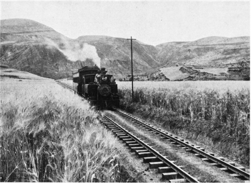
CENTRAL OF PERU RAILWAY, AYACUCHO VALLEY, 10,500 FEET
