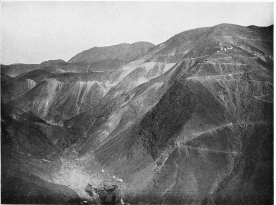
ARICA-LA PAZ RAILWAY WORKS AT ENTRANCE TO QUEBRADA PUJIOS
