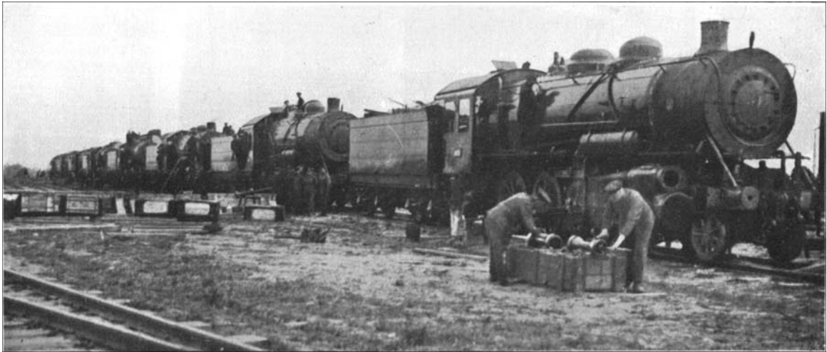
ERECTION OF BALDWIN ENGINES. FIG. 5.
