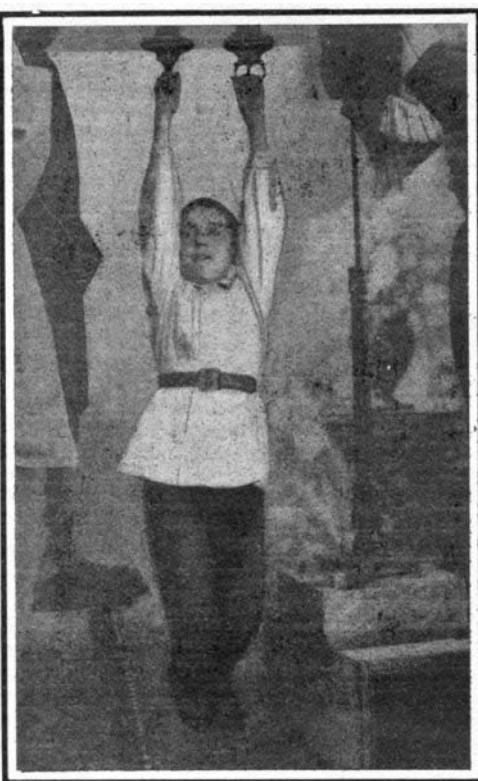
Disks Attached to Polished Surface, Supporting the Weight of a Boy.
