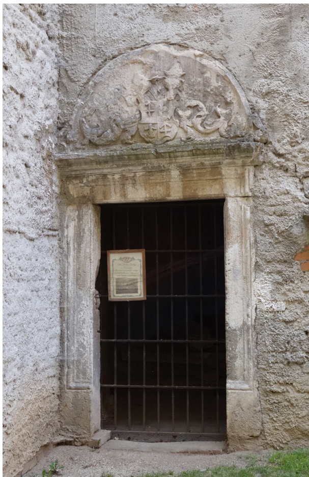
Figure 12: Portal on the courtyard, around 1540. Chateau in Dolní Kounice, Czech Republic. Source: Author's photo.
