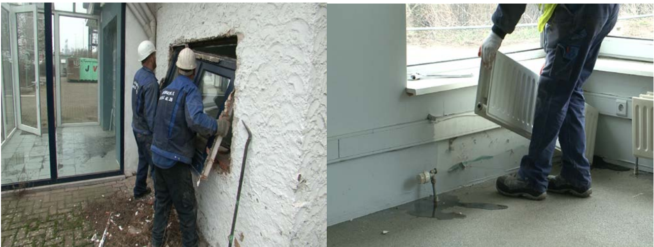
Figure 2: Dismantling of the materials that are suitable for reuse.
