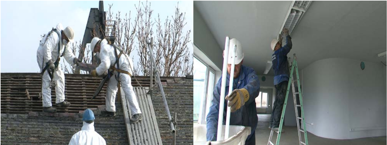
Figure 3: Decontamination of the building.
