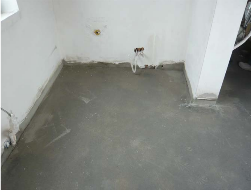
Figure 9: The installed floor screed with recycled AAC in the case study.
