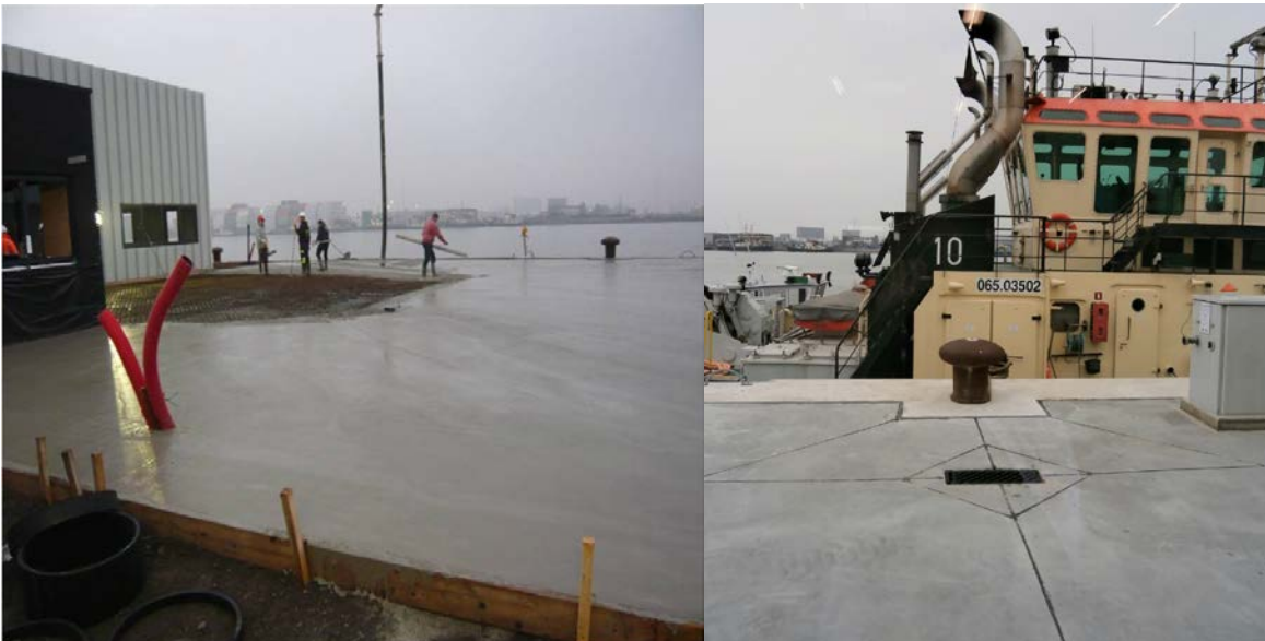
Figure 7: Polished concrete with recycled concrete aggregates in the PoA (left: during construction, right: user-phase).
