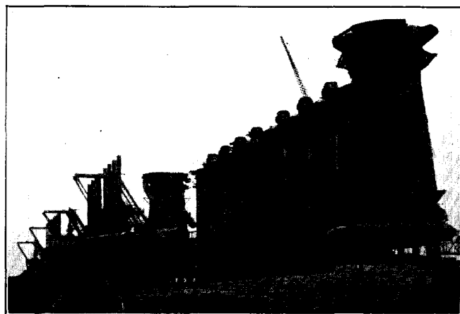
Fig. 9.—Blast furnaces and stoves under construction.
