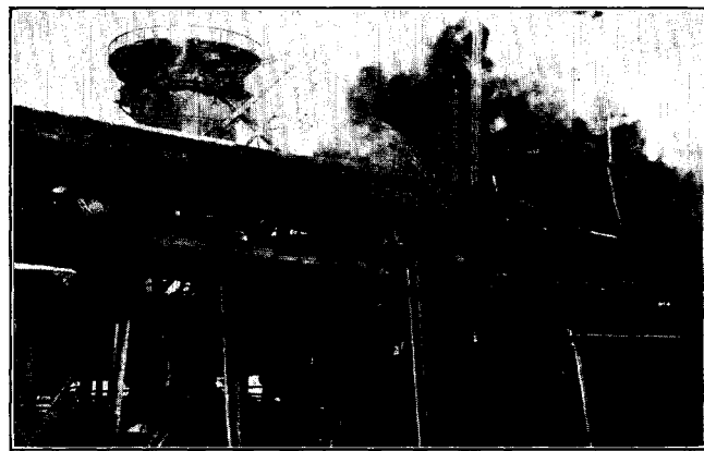
Fig. 14.—Back of blast furnaces. Gas mains leading to boiler house and secondary gas washers. Compliments of Allis-Chalmers Co.
