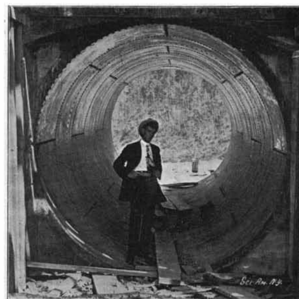
INSIDE PENSTOCK—9 FEET IN DIAMETER.
